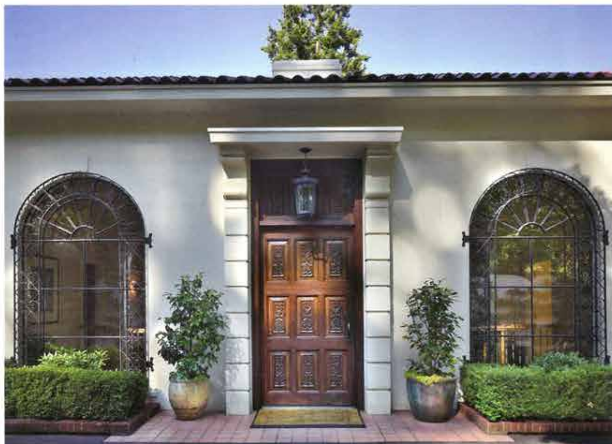
Above: The formerly pink and green exterior was re-stuccoed and painted a more neutral color. Right: Architect Tyler Engle and builder Owen Roberts revived many of the exterior details, refinishing the antique Mexican door and the lantern above it.
